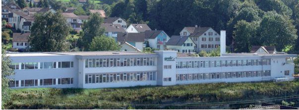
Our production site in Switzerland (Staad, SG)
