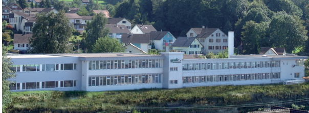
Our production site in Switzerland (Staad, SG)
